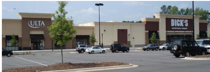
Roofline Variation and Parapet Finish
